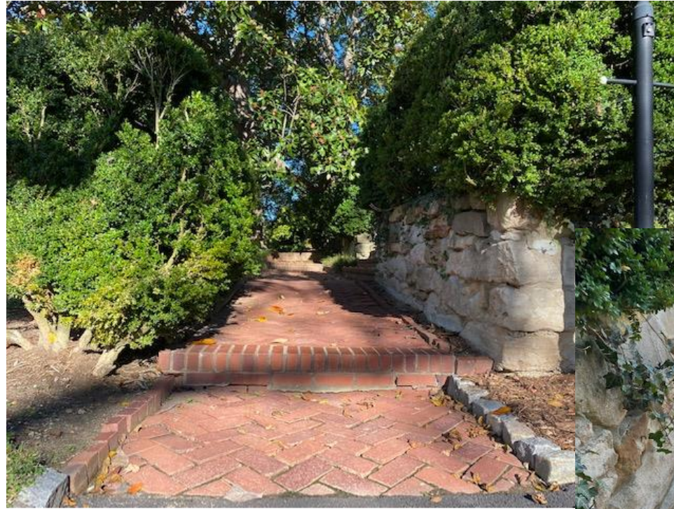
Rear walk to back patio, from parking (uneven transitions, settling; lift/grade/reset and mortar/polysand fill needed)
