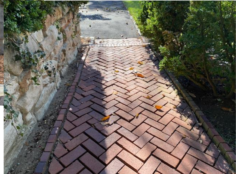
Rear walk to back patio, from parking (uneven transitions, settling; lift/grade/reset and mortar/polysand fill needed)
